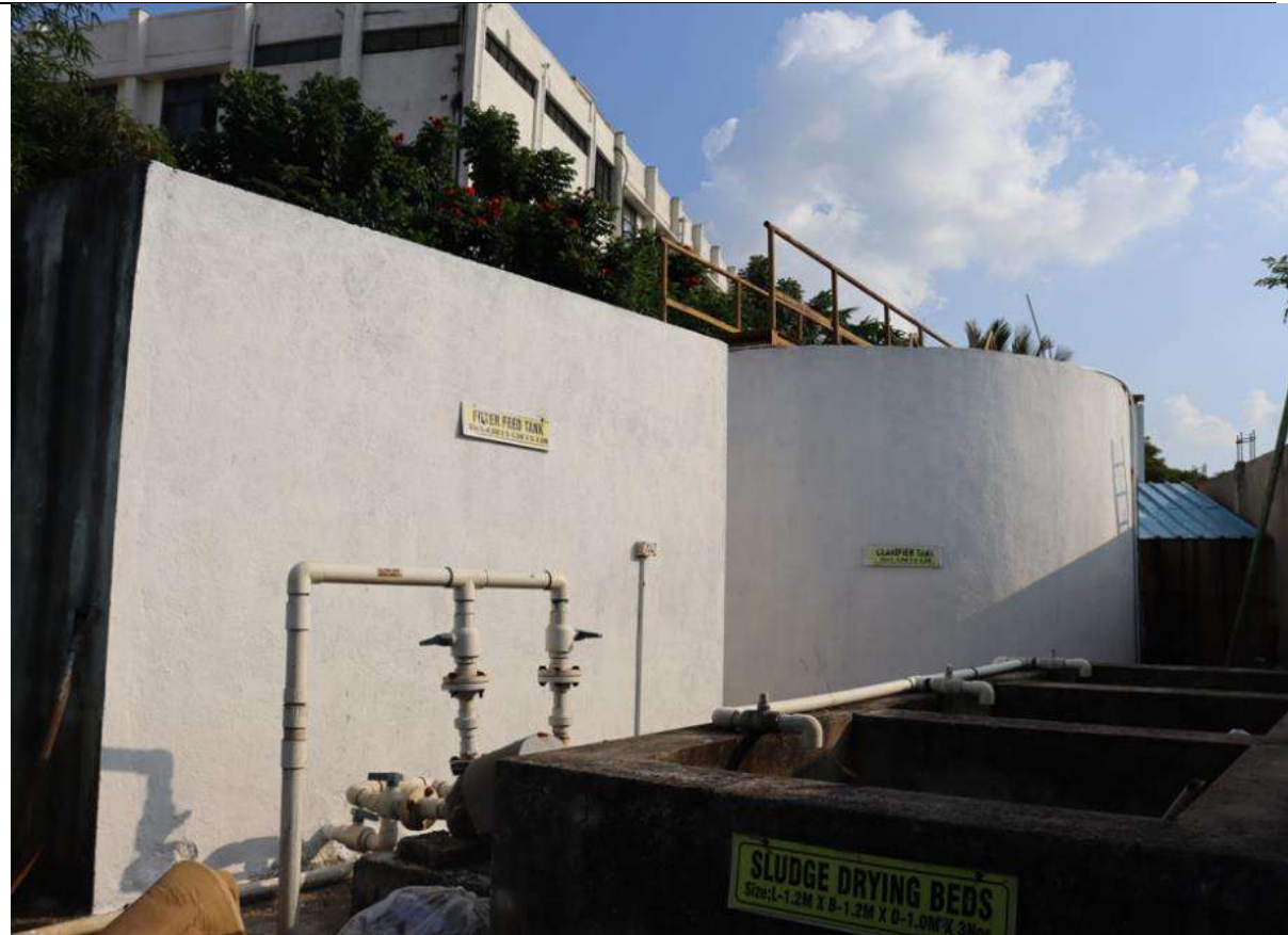
Filter Feed , Clarifier and Sludge drying Beds
