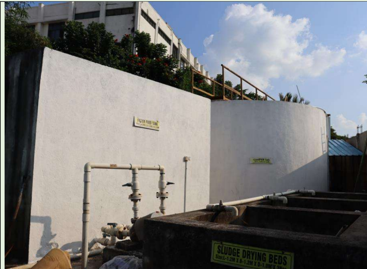
Filter Feed , Clarifier and Sludge drying Beds
