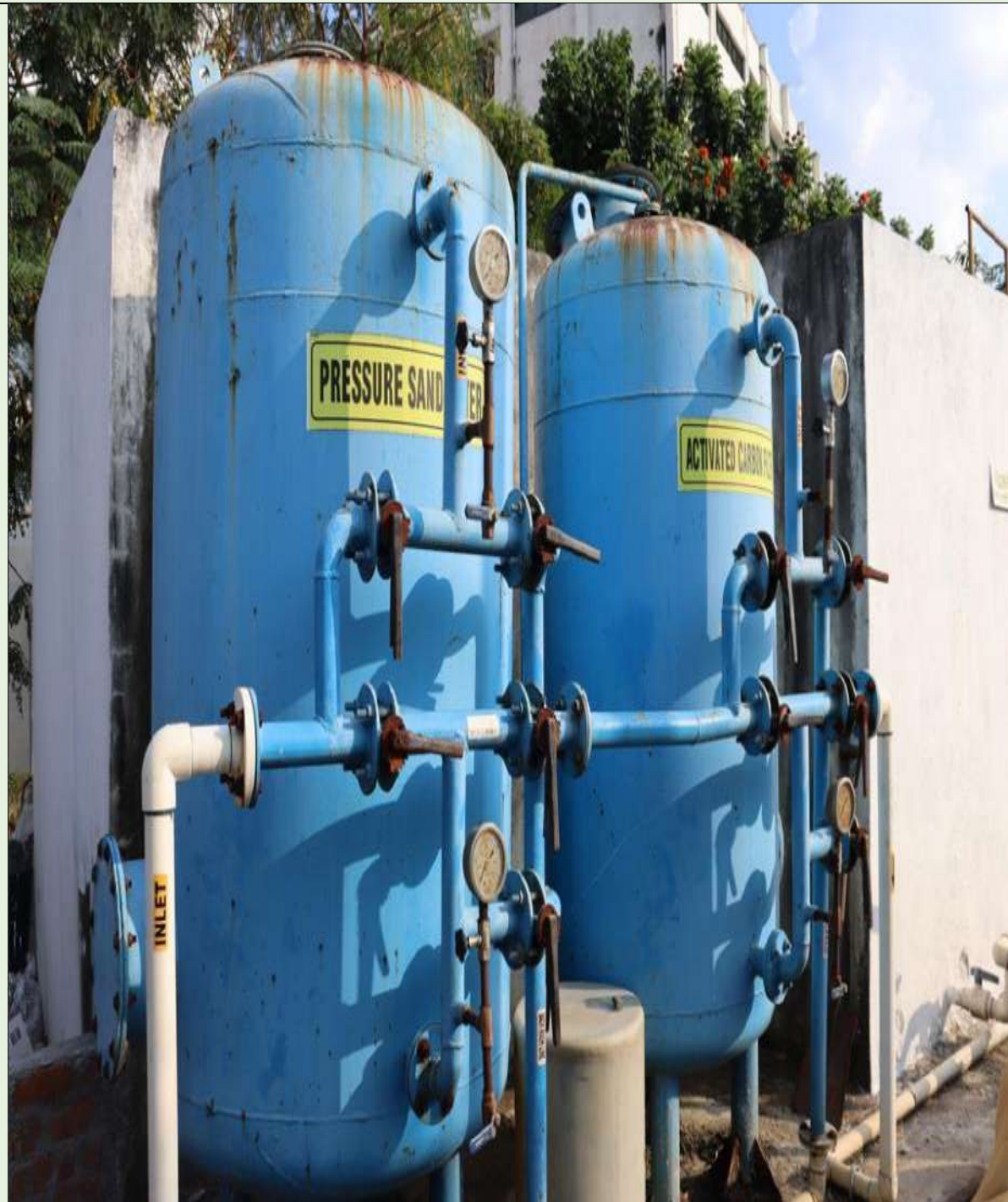
Pressure Filter Units
