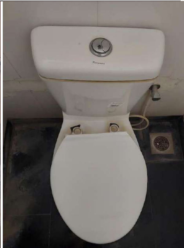
Dual-flush toilet tanks
