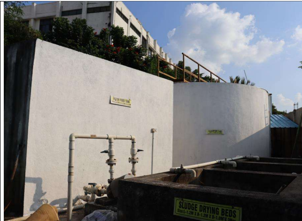
Filter Feed, Clarifier and Sludge drying Beds
