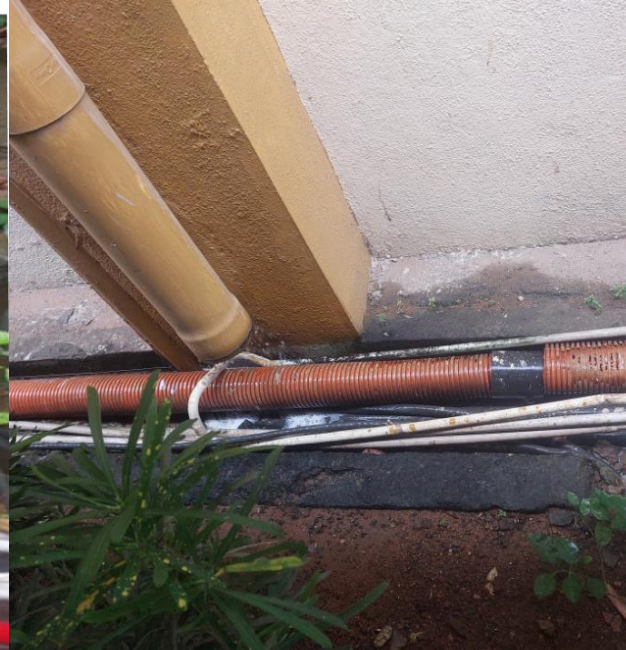
Different Colors of Pipes for Easy Maintenance
