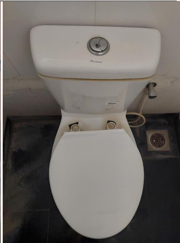
Dual-flush toilet tanks
