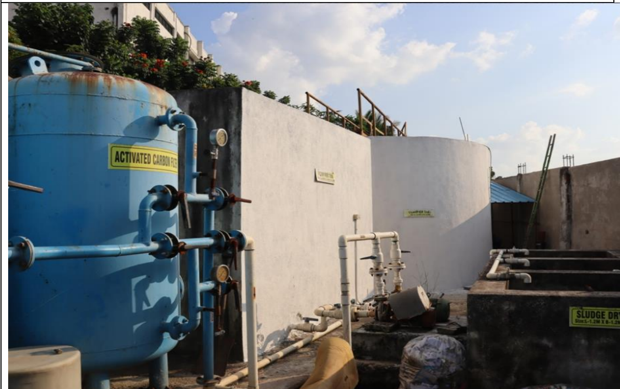
Pressure Filter Units
