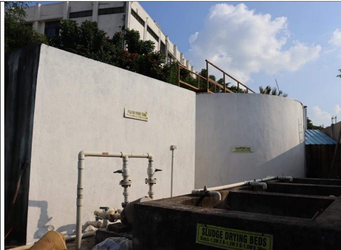
Filter Feed, Clarifier and Sludge drying Beds
