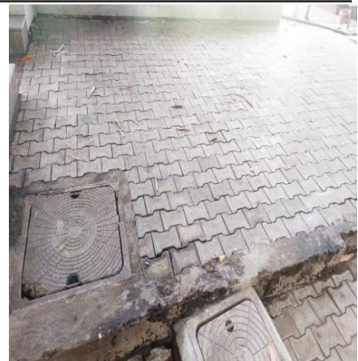
Ground Water Tank
