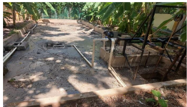
Waste Water Tank
