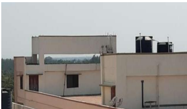
Clean Water Tank
