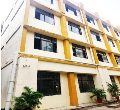
Rainwater Harvesting (Pipes)
