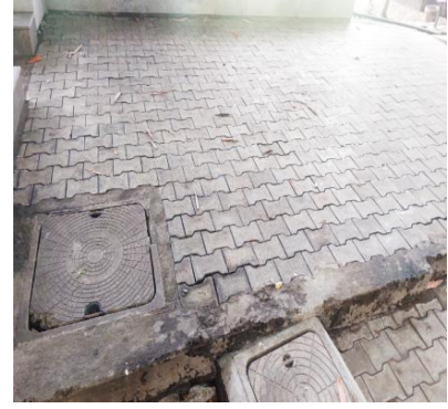
Ground Water Tank
