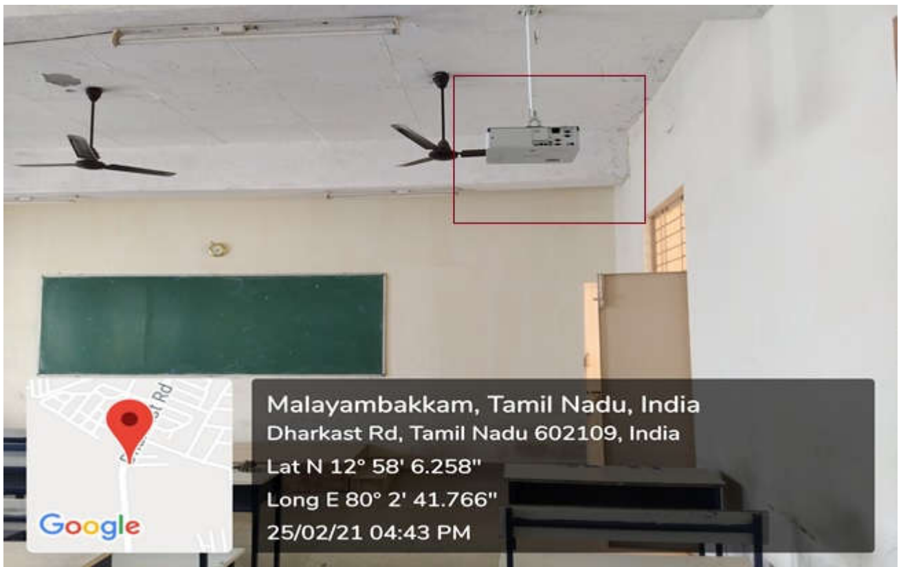
T12 Classroom inside view
