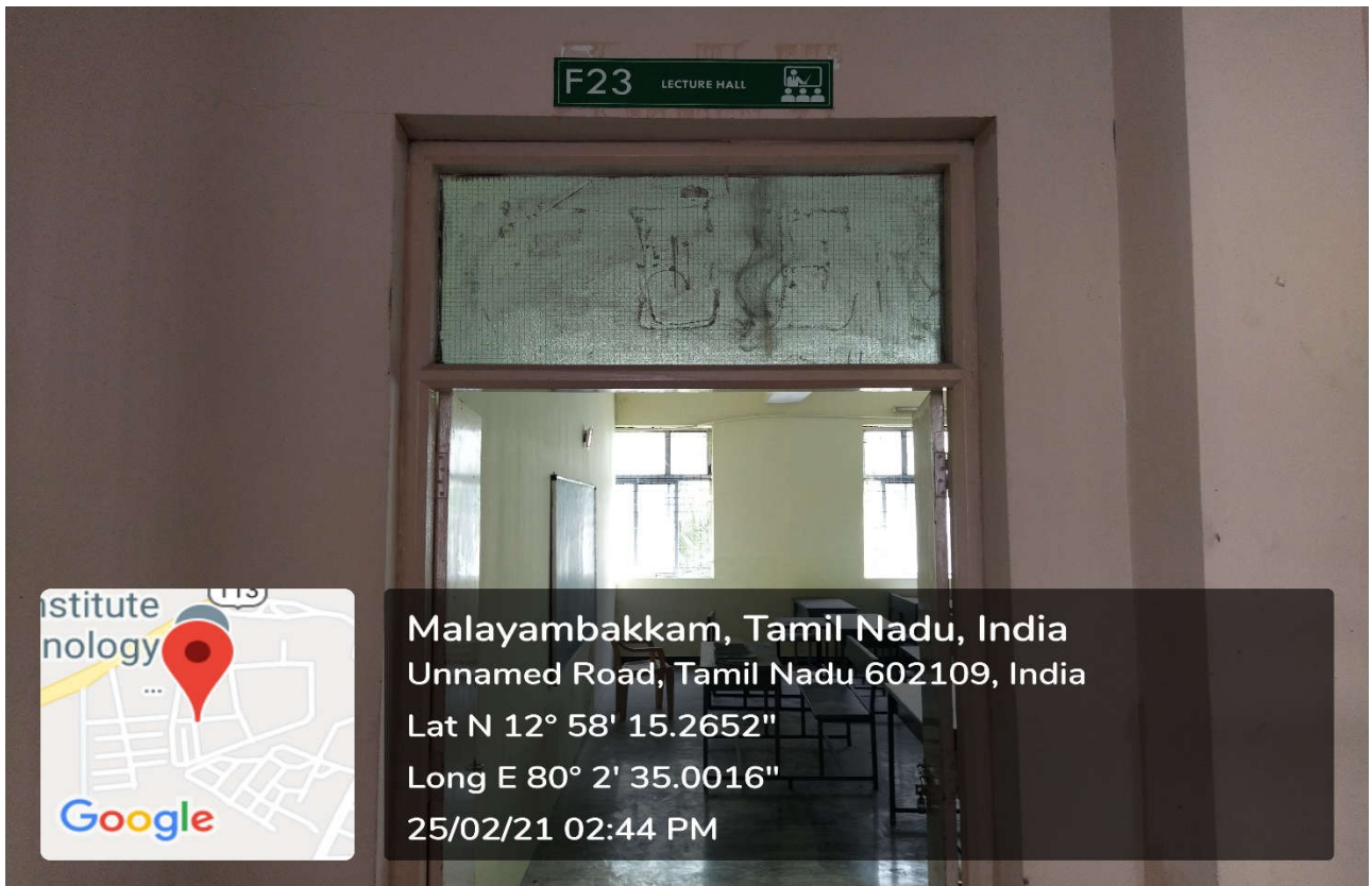
F23 Classroom outside view
