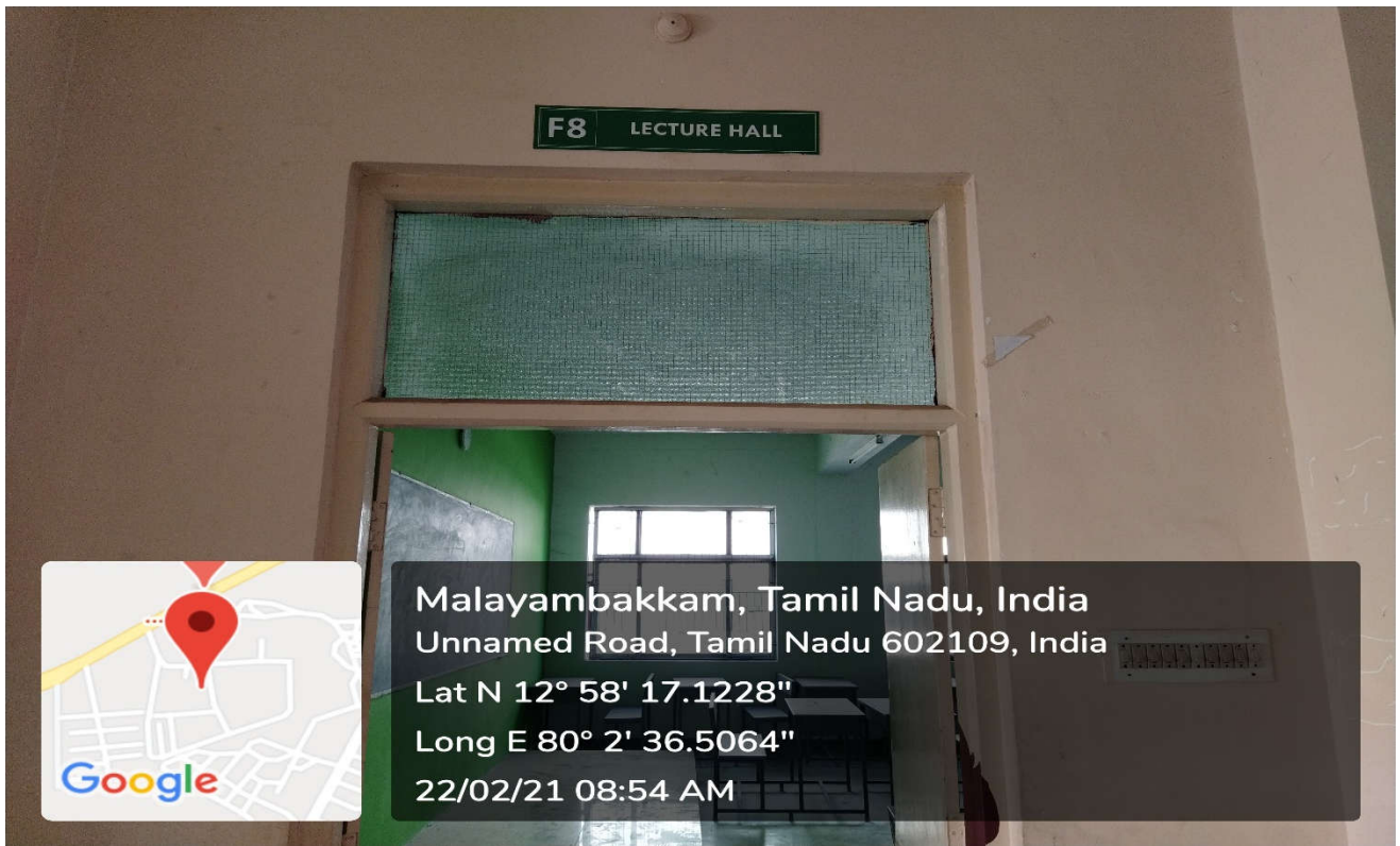
F8 Classroom outside view
