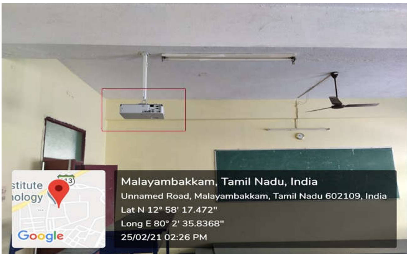
S5 Classroom inside view
