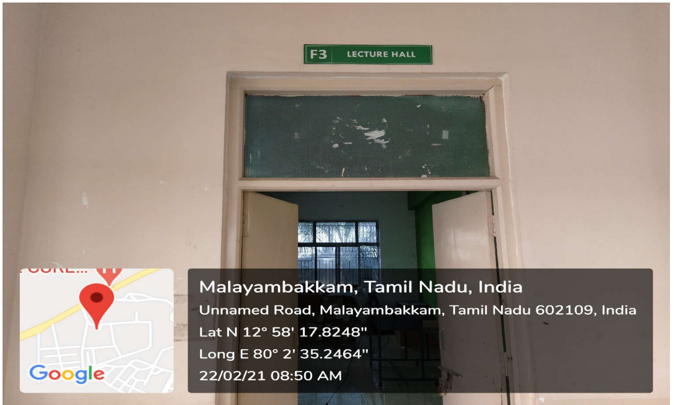
F3 Classroom outside view
