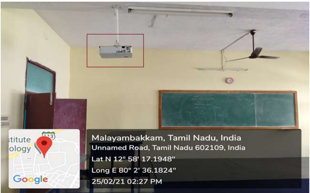
S6 Classroom inside view
