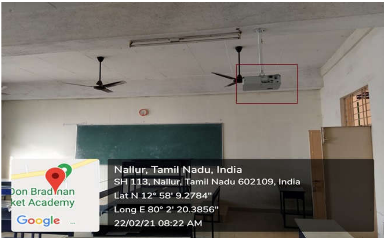
T20 Classroom inside view
