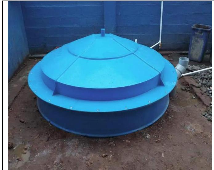
**Biogas plant – 100 kg capacity**
